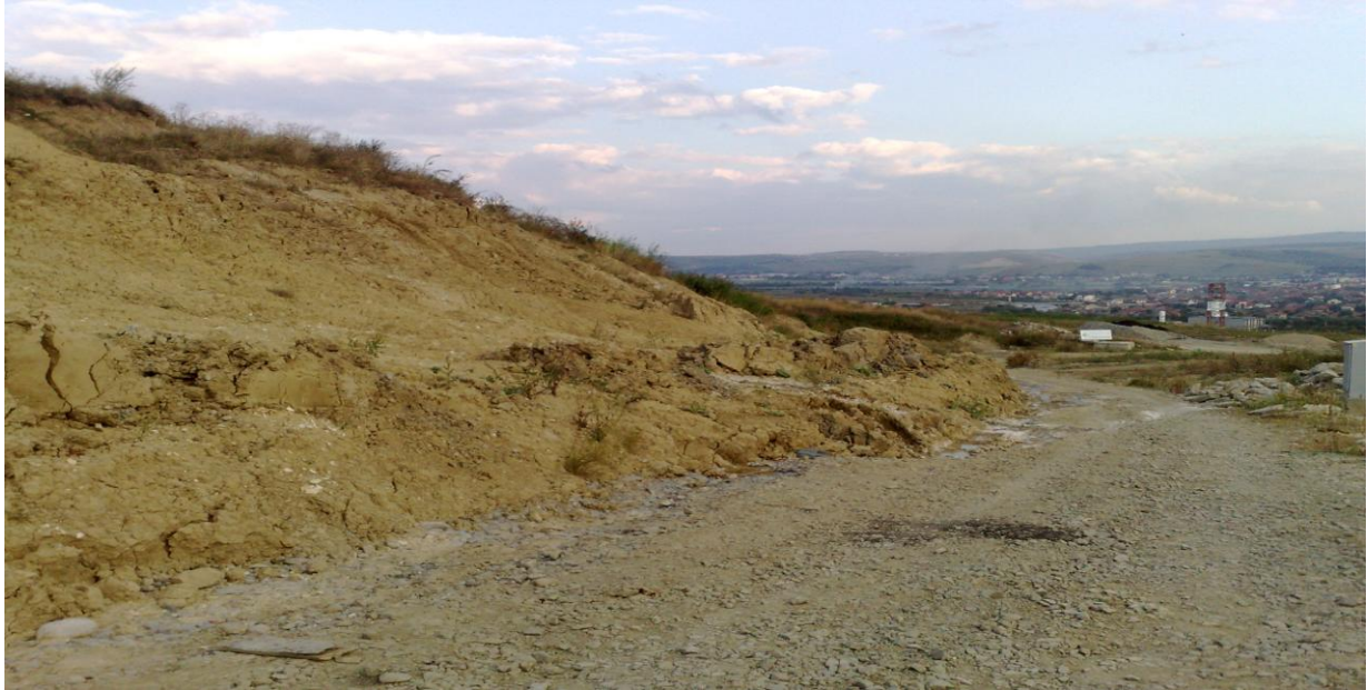
Fig. 3. Landslide caused by expansion of the road (southern slope of the hill Chinteni)
