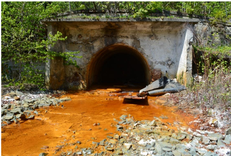
Figure 5. Entering the Breiner mine. (Doroțan Dora, May 2020)
