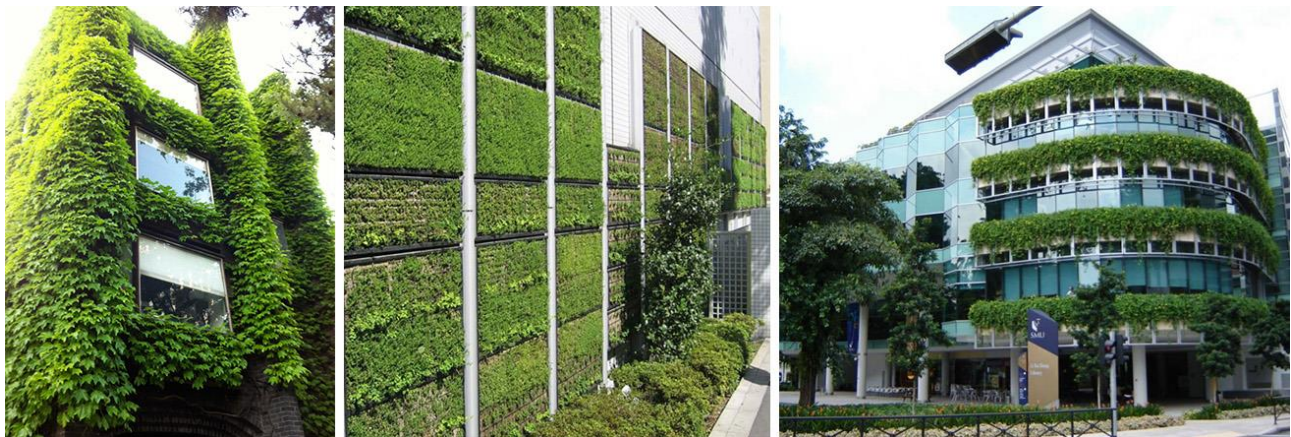
Figure 6.3 Traditional green facade, modular green walls and perimeter flowerpots; Source: www.static1.squarespace.com ; www.souceable.net ; www.lksf.org
