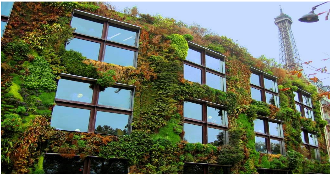
Figure 6.2 Vertical garden designed by Patrick Blanc at Museum Quai De Branly, Paris. Source: http://www.i.pinimg.com
