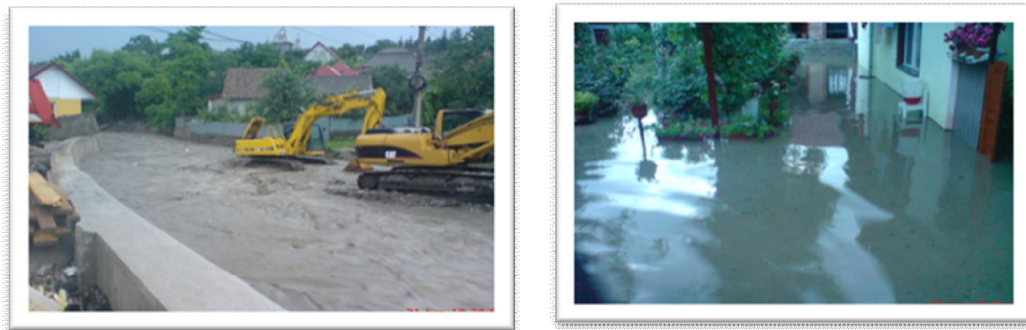
Fig.15. Racilor Valley overflowing, together with pluvial flooding in June 2010
