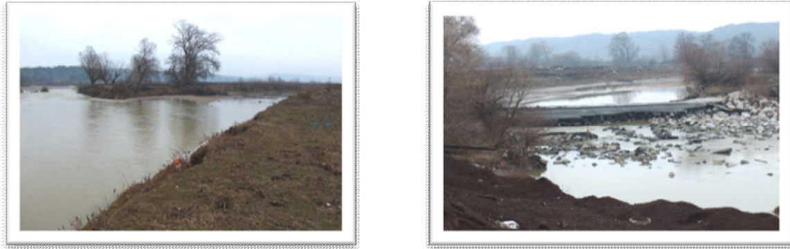
Fig.14. Arieș river deflected after the flood from December 2009 and the flooding flap of Mechel Factory
