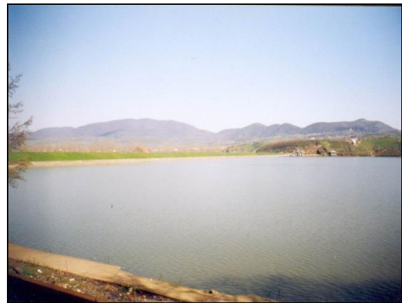
Accumulation lake – view towards dam
