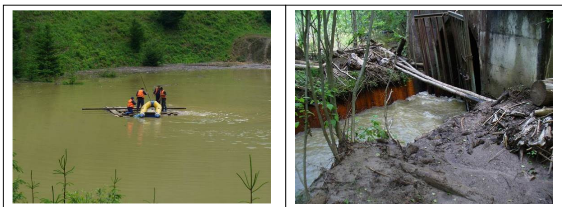
Fig. 11 Temporary lake formed on the top of the tailing dam endangering the downstream inhabitants and tourists located in Ostra village, and Fig. 12: detail of the diverting tunnel of the creek from the upstream area of the tailing dam, partially blocked with debris)
