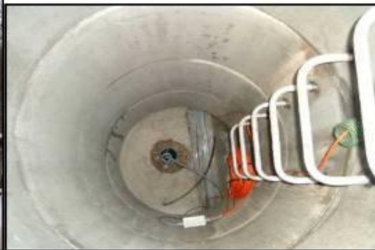
Figure 6.2 Visit chamber lever drain with sensor
