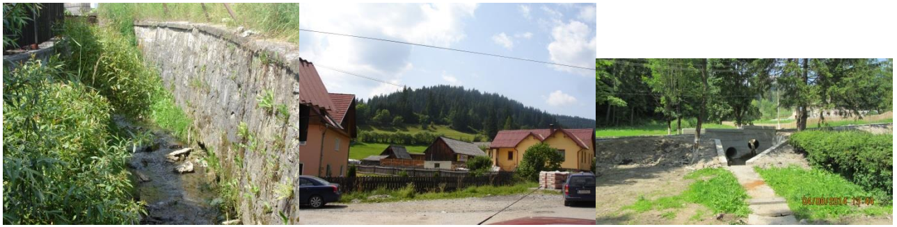
Figure 10.a. Brook bank reinforced.
