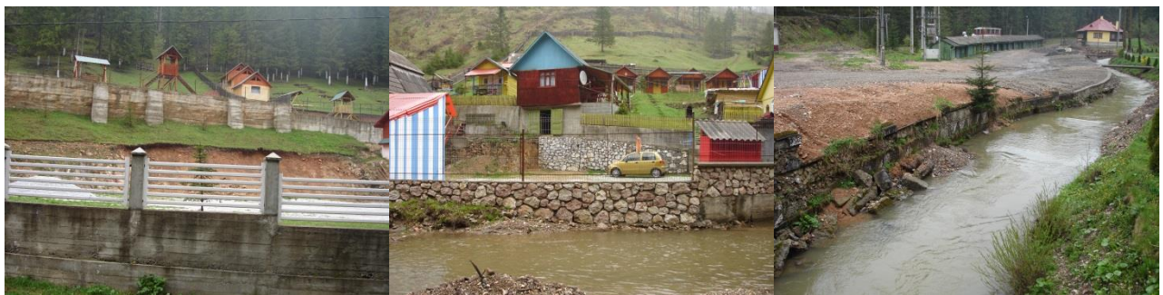
Figure 12. a. Constructing on terraces consolidated with concrete walls b. accommodation unit on the Oii valley c. Reinforced riverbed along the Bicaz
