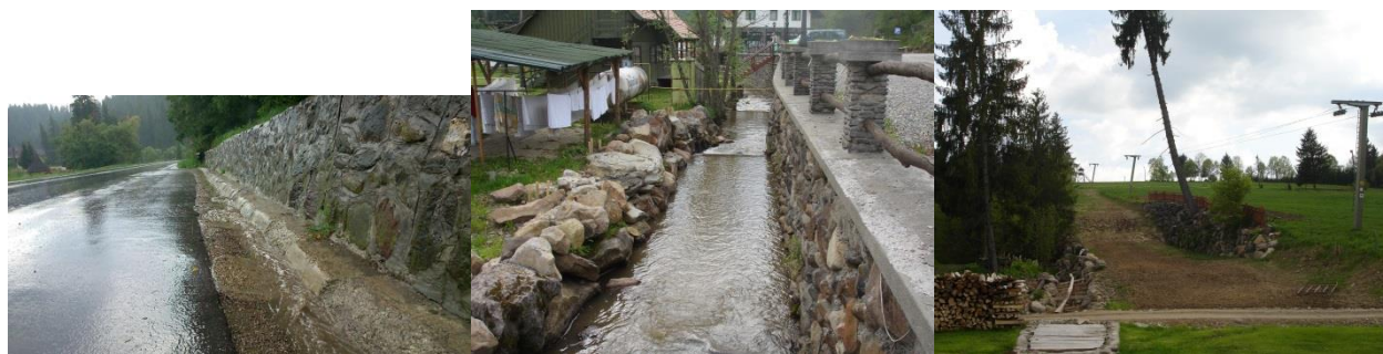
Figure 14 Adaptation to torrential downpours. a. Water course management on Homorodul Mic b. Brook management along the skirun Lobogo
