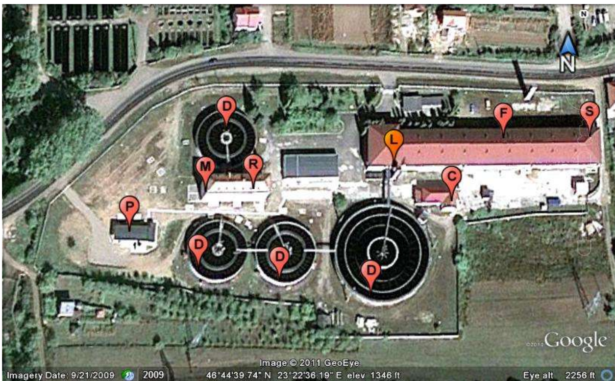
Fig. 2. Drinking water treatment process in Cluj: M – microstraining; P – prechlorination; R – reagents addition; D – clarification ; F – rapid sand filtration; C –final disinfection by chlorination; S – storage in reservoirs; L – laboratory.
