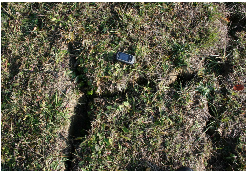
Foto 7.3. Polygonal cracks up to 10 cm wide, caused by the constraction of the silty clay (Baia Sprie, November 2012).
