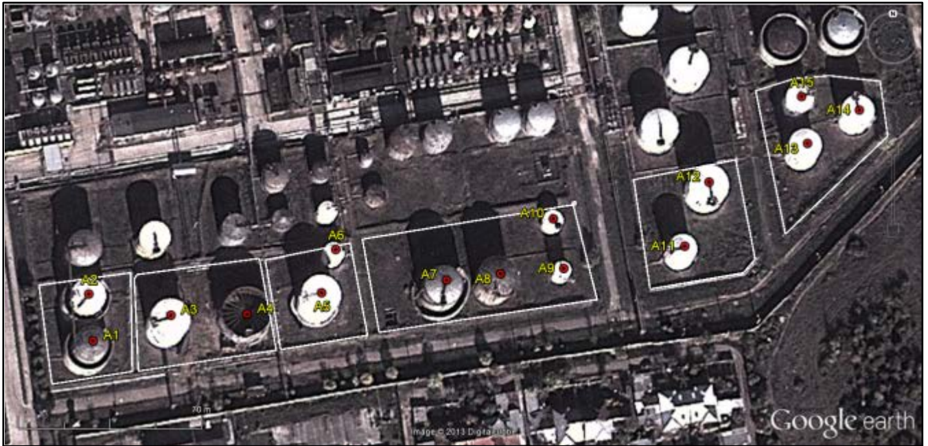
Figure 9. Tanks selected for the case study and the respective bund contours.
